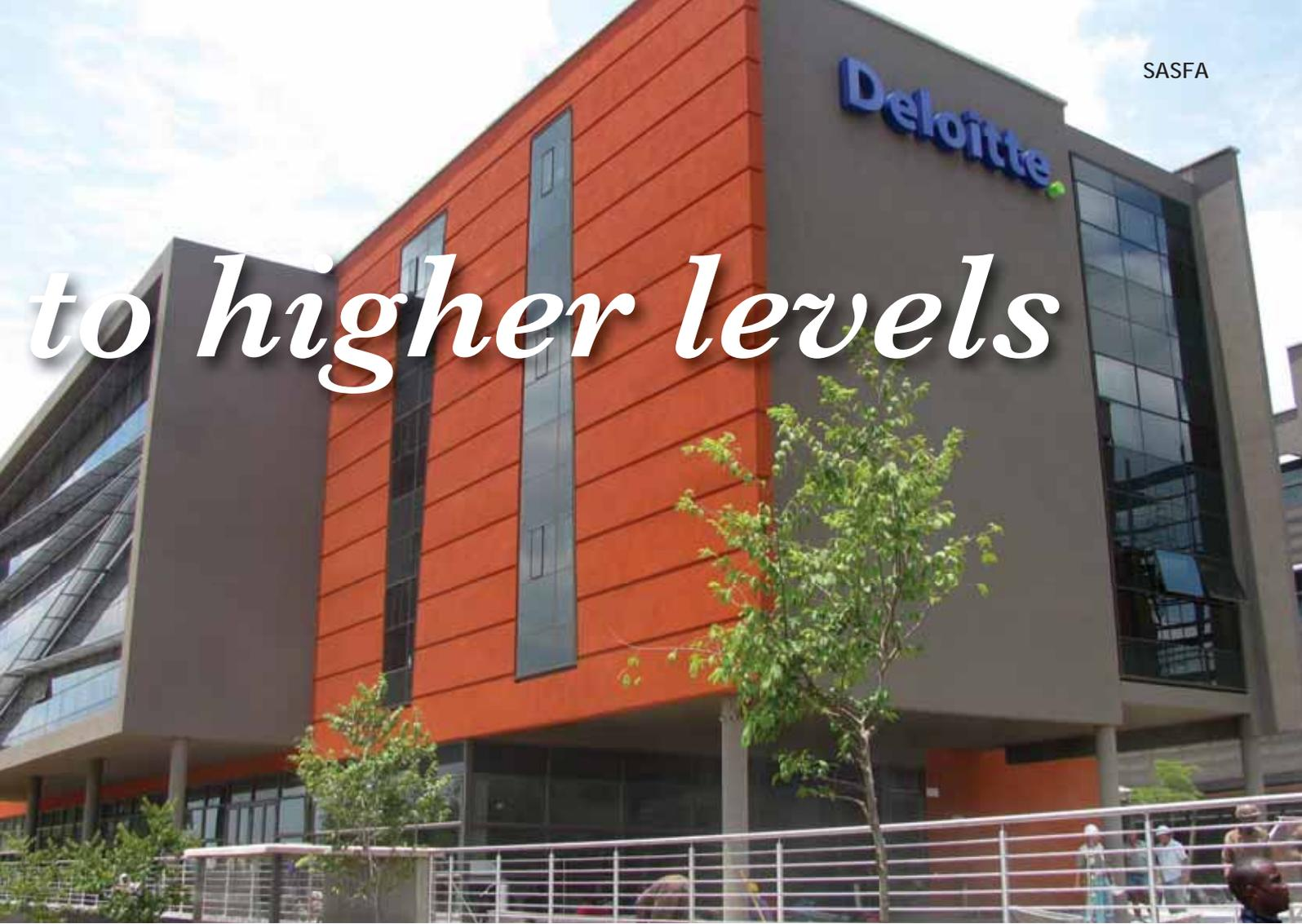
fixed. The external finish of the EPS consists of two layers of a special colour impregnated polymeric plaster. A reinforcing fibreglass mesh is embedded in the coating. This cladding system is referred to as EIFS (external insulating and finishing system). The inside of the light steel frames is clad with fire-resistant gypsum board. Additional insulation can be installed in the wall cavity, if required.
